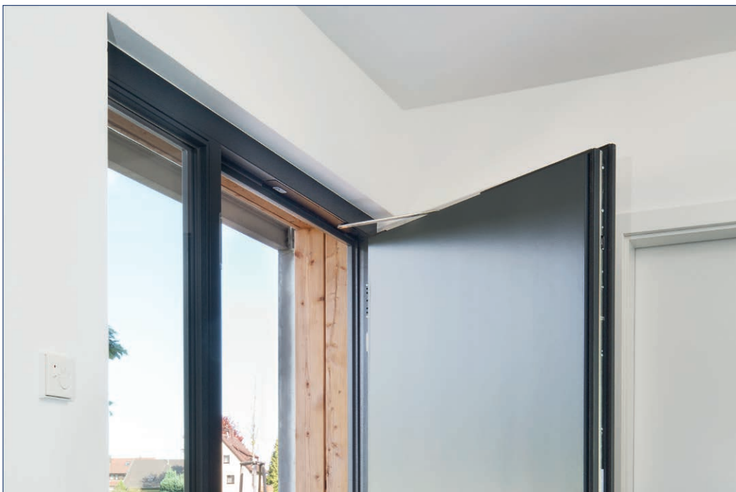
Entry door, private home, Stuttgart, Germany (Photo: GEZE GmbH)
