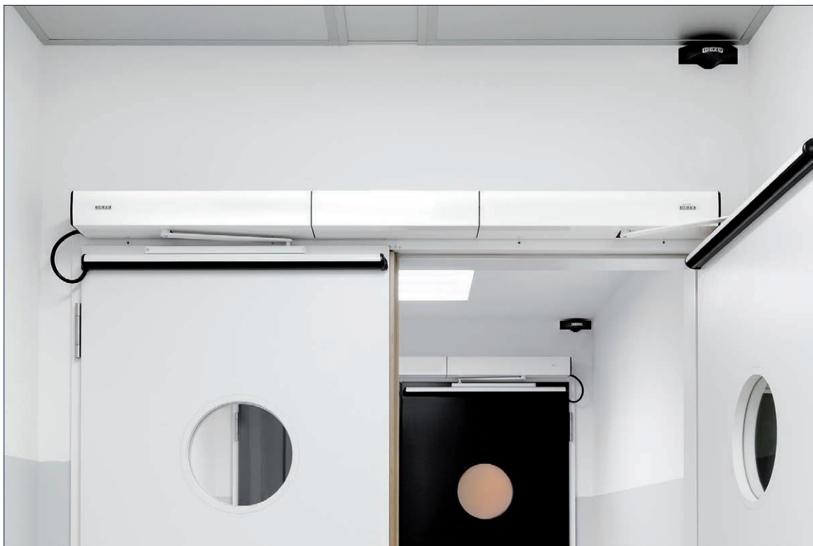
GEZE TSA 160 NT IS and radar movement detector, Andels Hotel, Berlin, Germany (Photo: Stefan Dauth)
