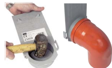
Removing knockout panel Pipe connection to endcap
