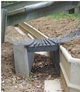
Stop Channel showing alignment with Guide Wall.
