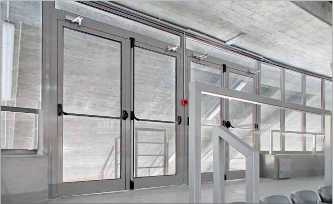
Sports Hall, Zadar, Croatia (Photo: Robert Les)
