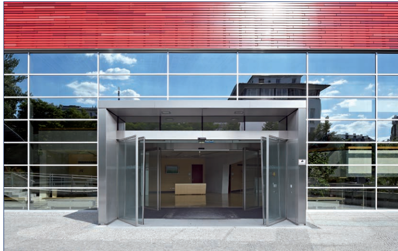
Rechts der Isar Hospital of the Technical University of Munich, Germany (Photo: Robert Sprang)
