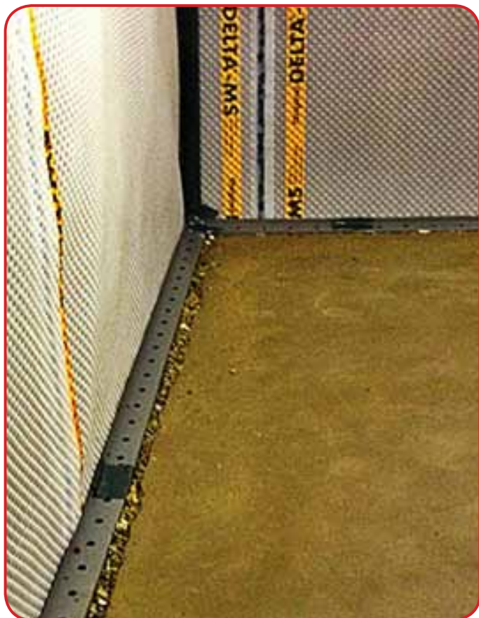
Typical 'Perimeter Channel' installation
