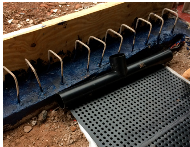
The steel intense ring beam was treated with Triton TT Vapour Membrane which easily copes around difficult details before the TGS-HP750 was sealed to it to create a fully sealed system
