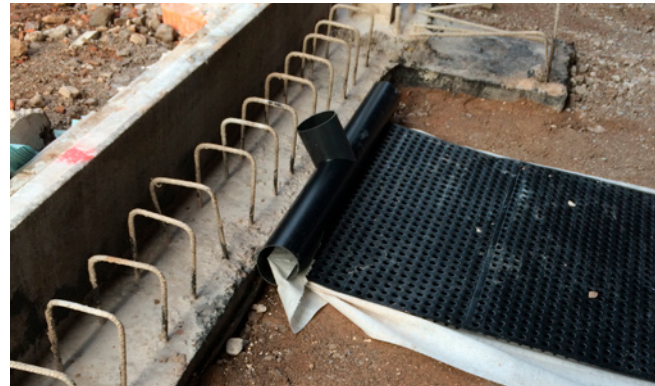
TGS-GV25 provides a void beneath floor slabs which, when connected to air inlets and outlets, allows sufficient air changes to dilute gases to safe concentrations
