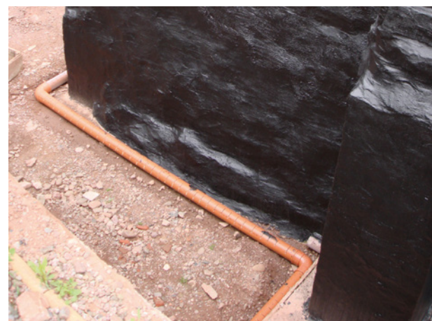
Triton TT Vapour Membrane to external walls
