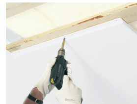
Focus F is installed by screw fixing
