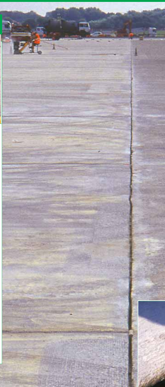
Linate airport - Milan - Italy Sealing of the runway joints with: MAPEFLEX PB27
