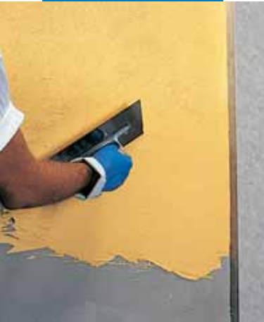
Applying Silexcolor Tonachino with a trowel
