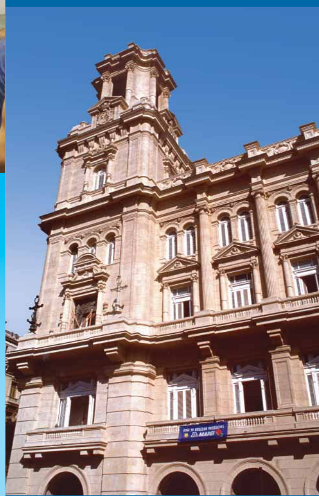
Asturian Centre Building - Havana - Cuba Restoration and protection of the façades of the building using: MAPEGROUT THIXOTROPIC , MAPEFER , MAPE-ANTIQUE FC , MAPE-ANTIQUE MC , MAPE-ANTIQUE LC , SILEXCOLOR PAINT
