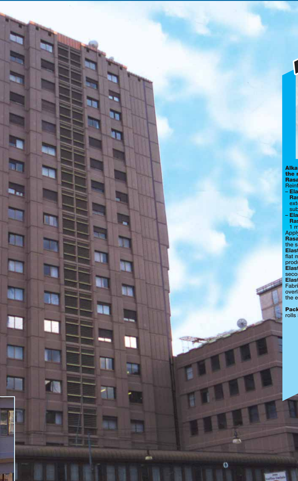
Reale Mutua Insurance building - Milan - Italy Restoration and protection of the façades of the building using: MAPEFER, MAPEGROUT BM, MALECH, ELASTOCOLOR RASANTE
