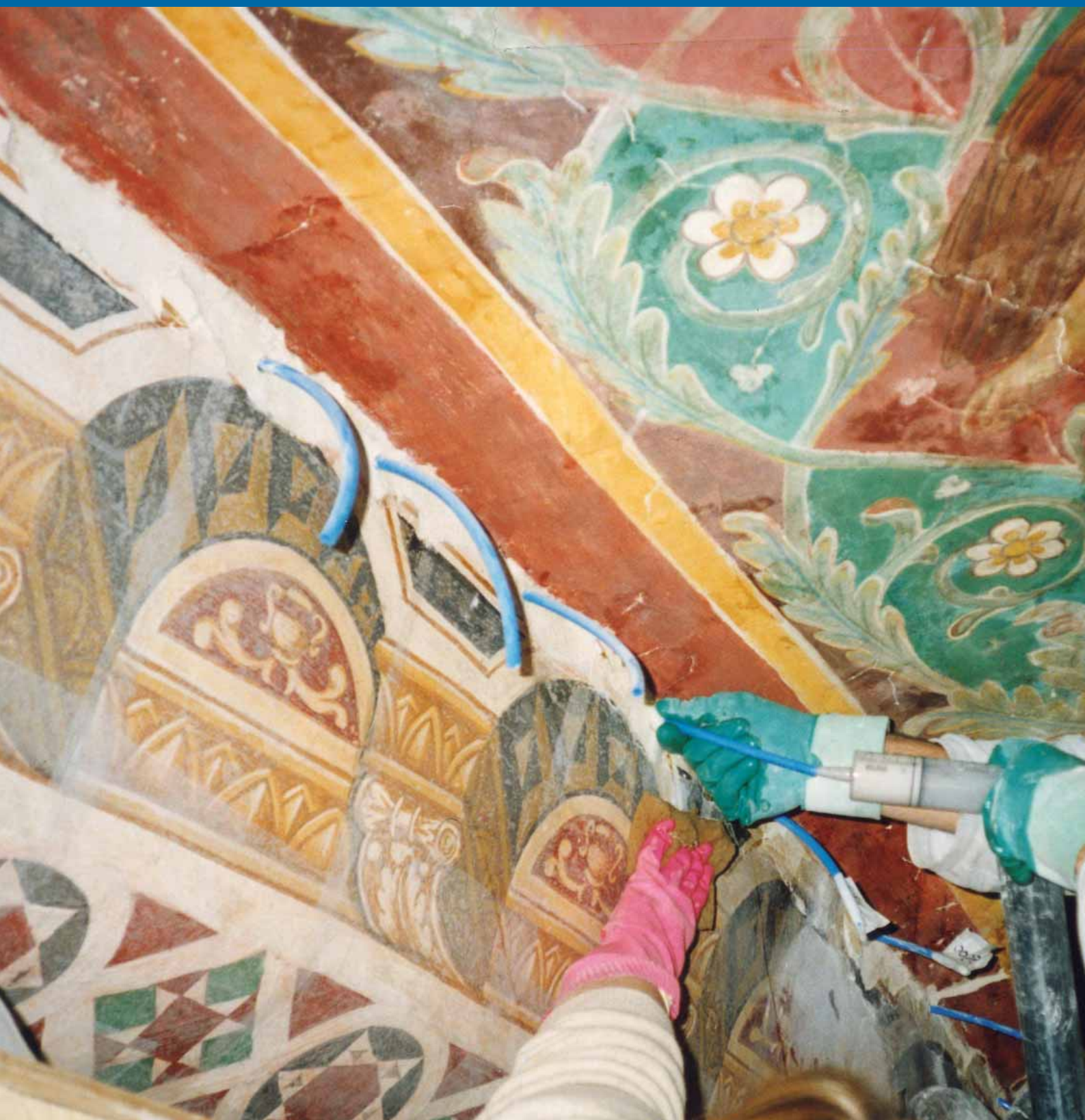
Basilica of San Francesco d'Assisi - Assisi - Italy Consolidation of the masonry using: MAPE-ANTIQUE I, MAPE-ANTIQUE F21
