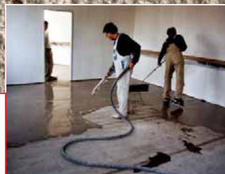
MAGNA STEYR GROUP PLANT - Graz - Vienna Substrate preparation with: NIVORAPID, ULTRAPLAN, PRIMER G. Installation of linoleum with AQUACOL T
