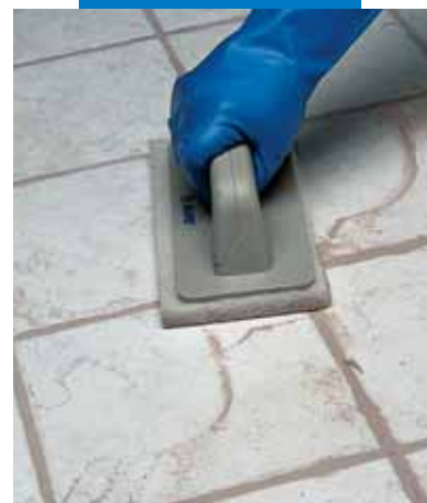
Finishing with a Scotch-Brite® pad
