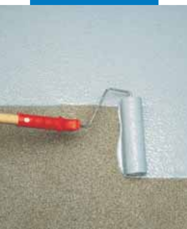
Applying Mapecoat I 24 with roller
