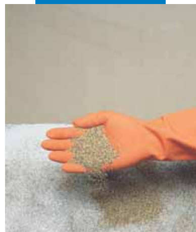
Spreading dry sand on fresh Mapecoat I 24
