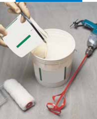
Mixing component B with component A
